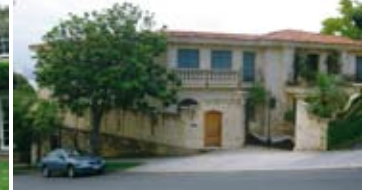
Q2. 63 Wolseley Road, Point Piper $21.5million
